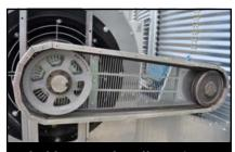
Belt-drive Operation offers quieter (3 dB less), smoother fan operation with less vibration compared to direct drive single inlet fans. It also makes drive system maintenance easy. The fan safety guard has been removed to show the belt drive in this photo.
