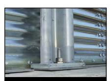
Anchor Rod/Bolt System is included on all models. The adhesive or cast-in anchors provided meet new ACI concrete code requirements and help create a strong, weathertight connection to the foundation, protecting your investment from winds up to 105 mph (169 kph).
