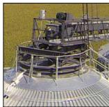
With Higher Bin Roof Peak Loading, it is crucial to safely transfer loads correctly and directly into the roof structure. The Brock EVERLOC® Roof Mount System's support components are attached directly to the roof structure during bin construction to ensure proper load transfers into the structure.
