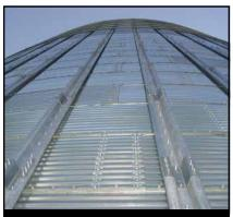
All-Galvanized Steel stiffener design carries 100% of the bin's vertical load stresses and leads the industry in strength. Stiffeners are assembled with bolt heads inside bin and flange nuts outside for easier assembly and to minimize interior grain hang up points.
