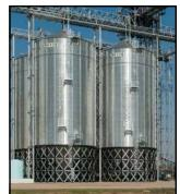
Steep Hopper Angles (up to 60°) aid the unloading of wet or dry whole kernel grains of many types.
