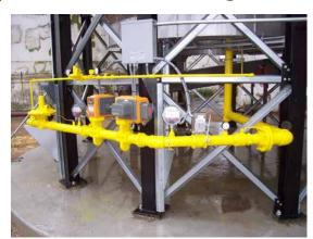
Commercial block and bleed gas train is standard with high & low gas safety pressure switches.
