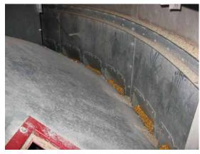
Brock's unique self-cleaning plenum floor design allows fines, dirt and bees' wings to recycle back into the grain safely while also reducing routine cleaning maintenance.
